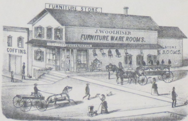
J. WOOLHISER COR. MADISON & DIVISION STS. BLDG. NO. 1114
